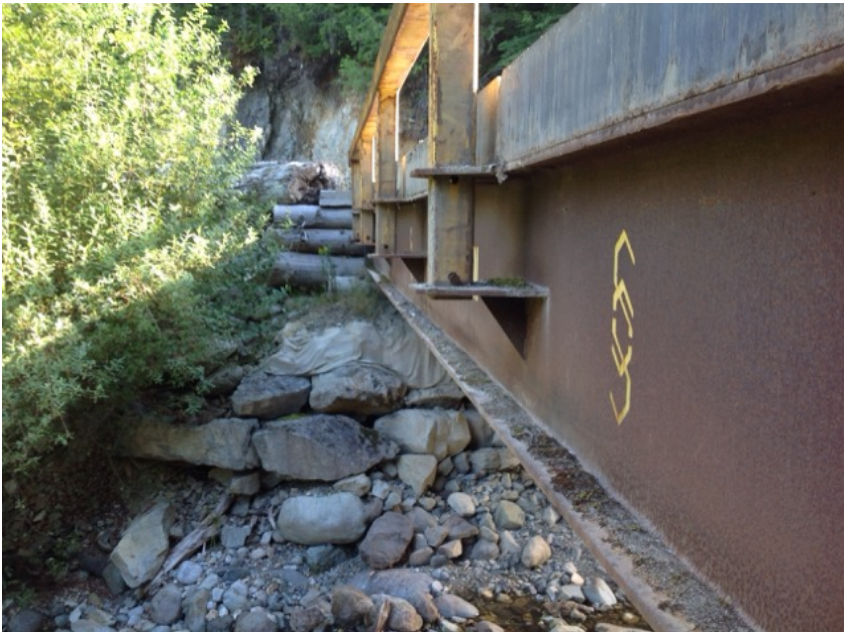
rail connection - slides down through steel plates
