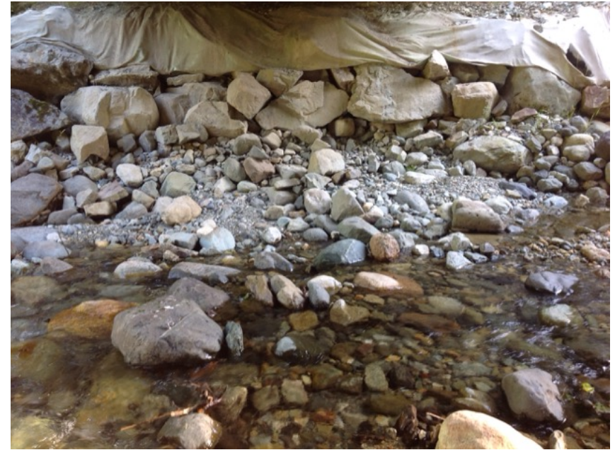
stream bottom approx 1.0m below bottom riprap elevation
