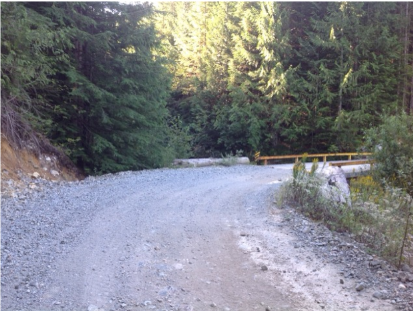
Approach from Right Bank when facing downstream
