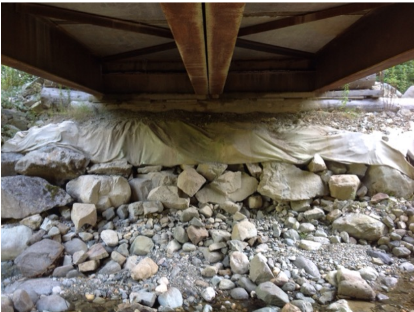
Right Bank Abutment when facing downstream
