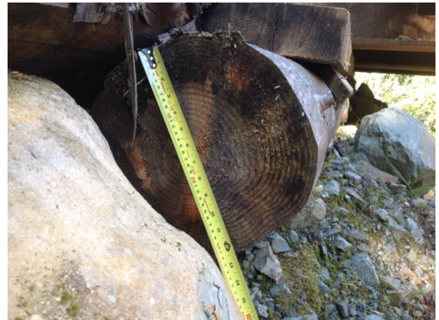
upstream log sill diameter
