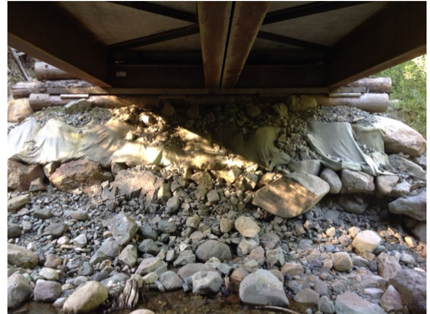
Left Bank Abutment when facing downstream
